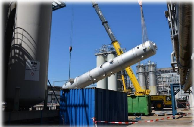
Destillationskolonne Ø 2400 x 22000mm
